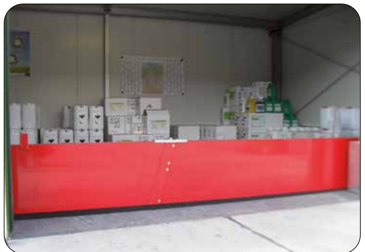
Firewater retention with rotating, hinged barrier
