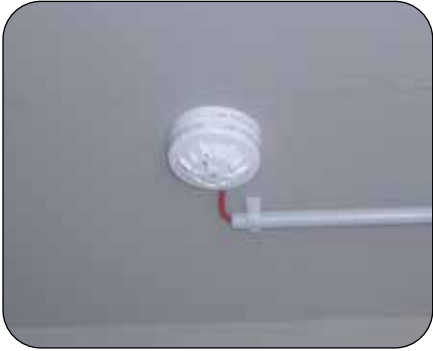
Heat detector for controlling the door locking system
