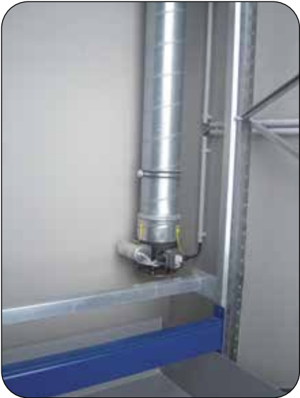
Exhaust air system including fire-protected ventilation elements
