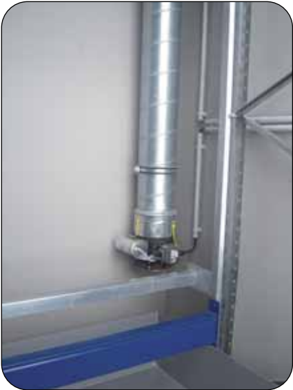
Exhaust air system including fire-protected ventilation elements
