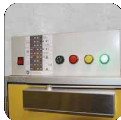
Control unit with fire detection
