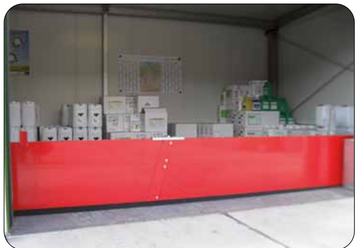
Firewater retention with rotating, hinged barrier
