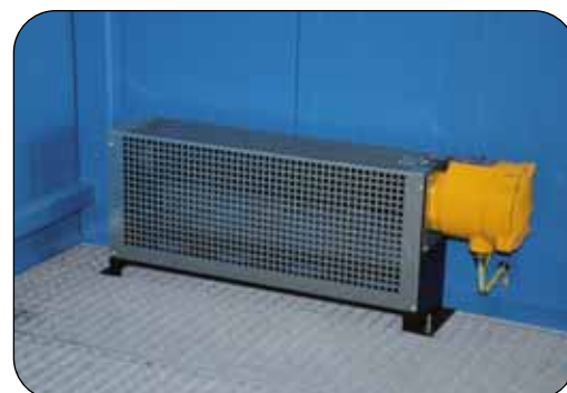
Ex-proofed heating 1,5 kW
