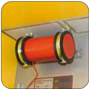
Aerosol extinguishing generator
