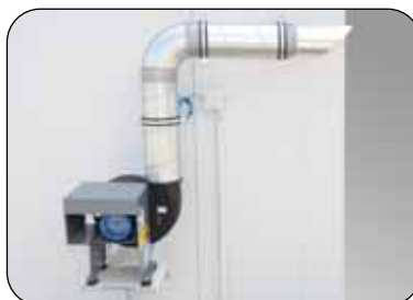
Ex-proof exhaust fan incl. exhaust air monitoring
