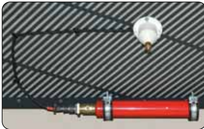
Aerosol extinguishing system
