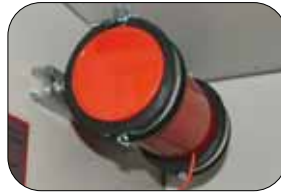
Aerosol extinguishing generator
