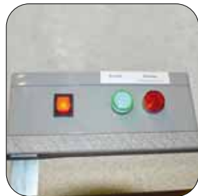
Control unit with smoke detection
