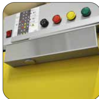
Automatic door closing device
