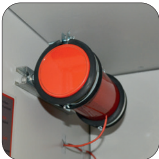
Aerosol extinguishing generator
