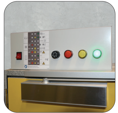
Control unit with fire detection
