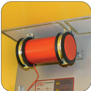
Aerosol extinguishing generator
