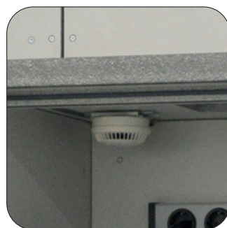
Integrated smoke detector
