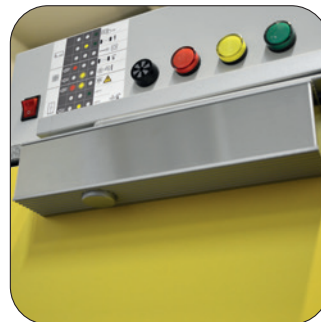
Automatic door closing device
