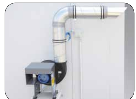
Ex-proof exhaust fan incl. exhaust air monitoring
