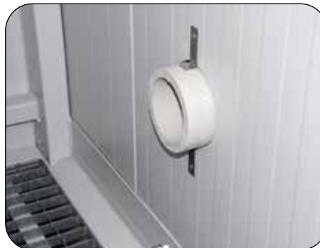
K-90 shut-off device
